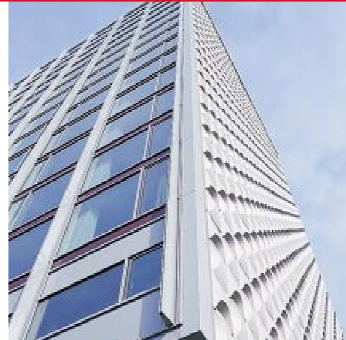
Hotel Mercure, Dresden, Renovation of façades WICTEC EL
